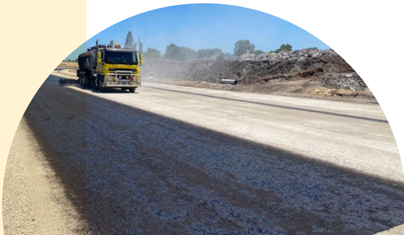
Photo: Main Roads WA
